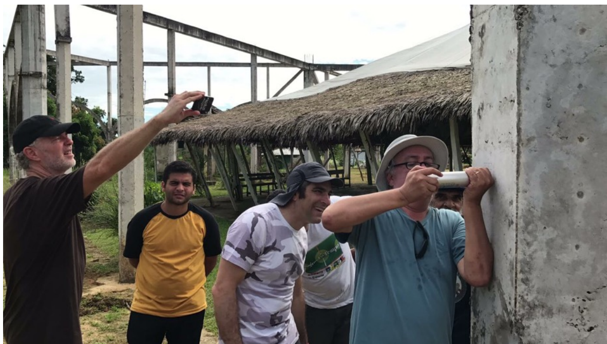
Engineers analyzing soil and foundations, and measuring concrete structure.
